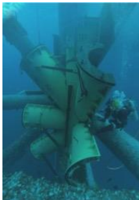
Installation of platform structure clamp
