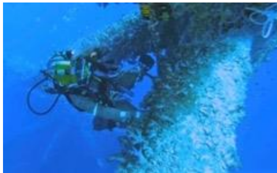
Diver conducting platform inspection
