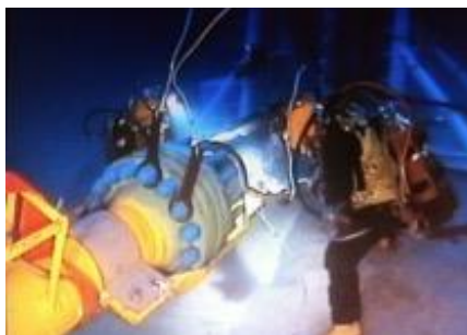
Spool installation by saturation divers
