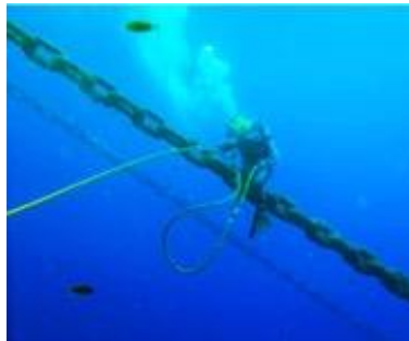
Diver inspecting mooring chain
